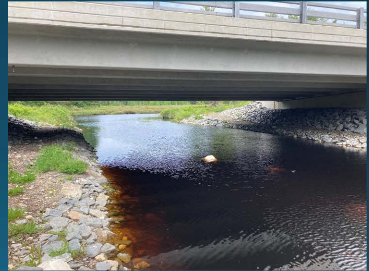
Replacement structure: 72' span bridge with internal wildlife shelves and improved habitat connectivity. Construction was completed in 2019.
