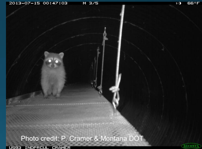
Montana's wildlife shelf in a culvert that conveys water
