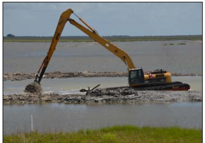
Specialized equipment called marsh buggies are used to build marsh terraces.
