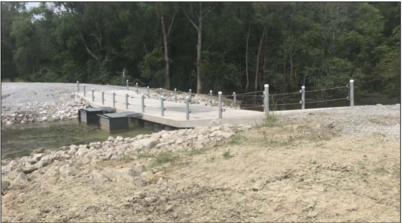
Pomme de Terre WMA. The addition of flashboard risers to the new weir structures gives LDWF better management capacity.
