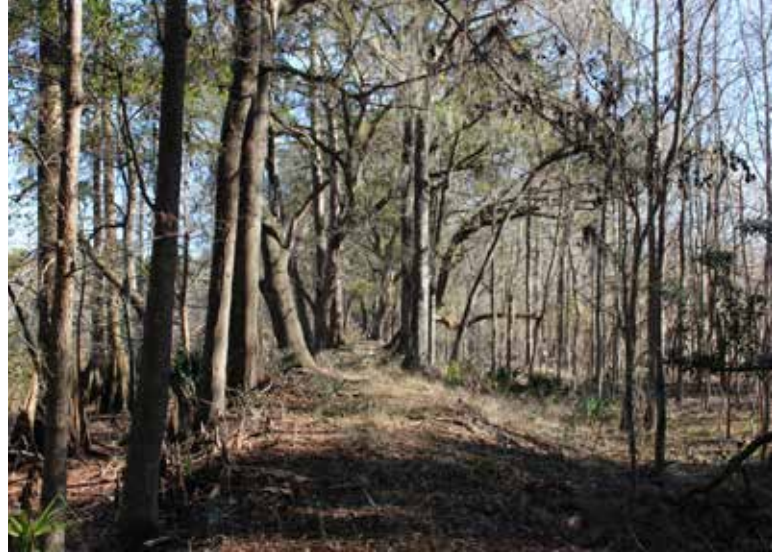
Before: Lake Emily embankments were dominated with trees and inadequate elevation for maximum capacity.
