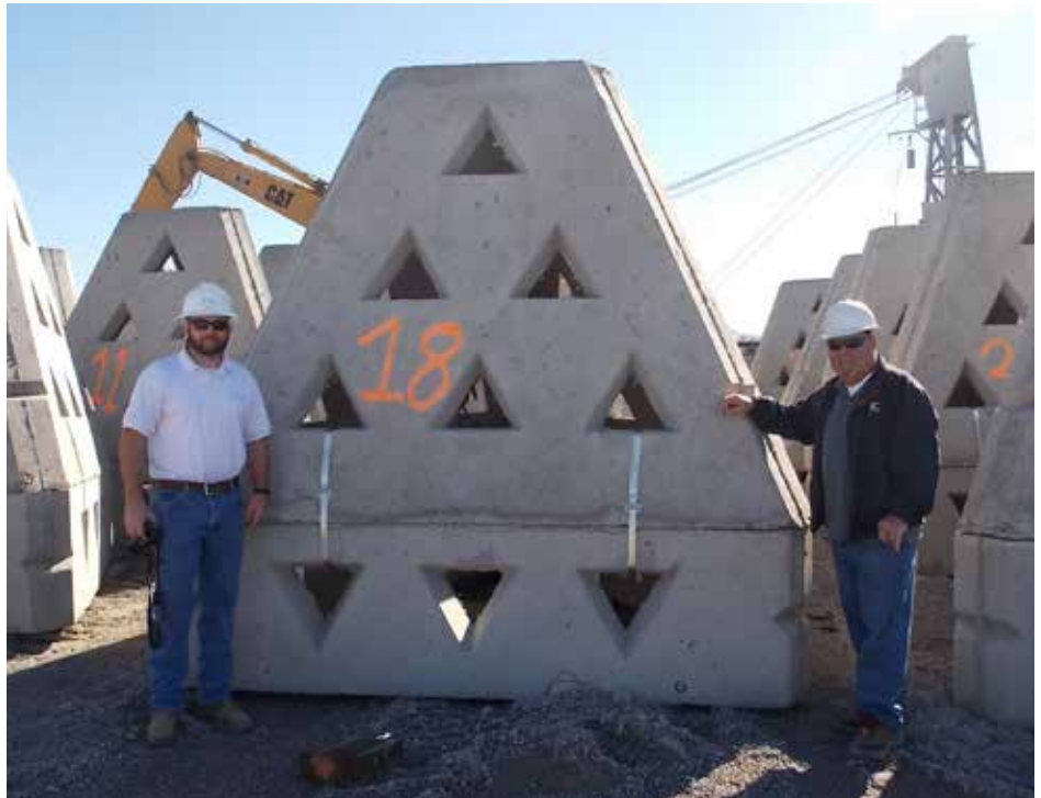
Living shoreline site visit 1.27.2015 036.jpg - DU Engineer Joe Fifer (l) with Sterling Robicheux of Low Land construction next to a wave attenuation device (WAD).
