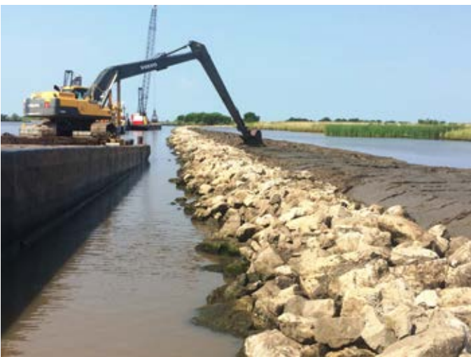
This breakwater will stabilize the shoreline along Freshwater Bayou and promote marsh growth.
