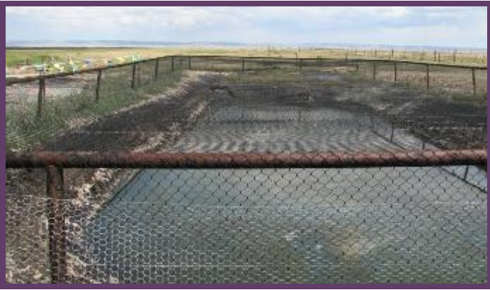
Netting appears to be the most effective method of excluding birds and other wildlife from entering waste pits containing produced water. Credit: USFWS
